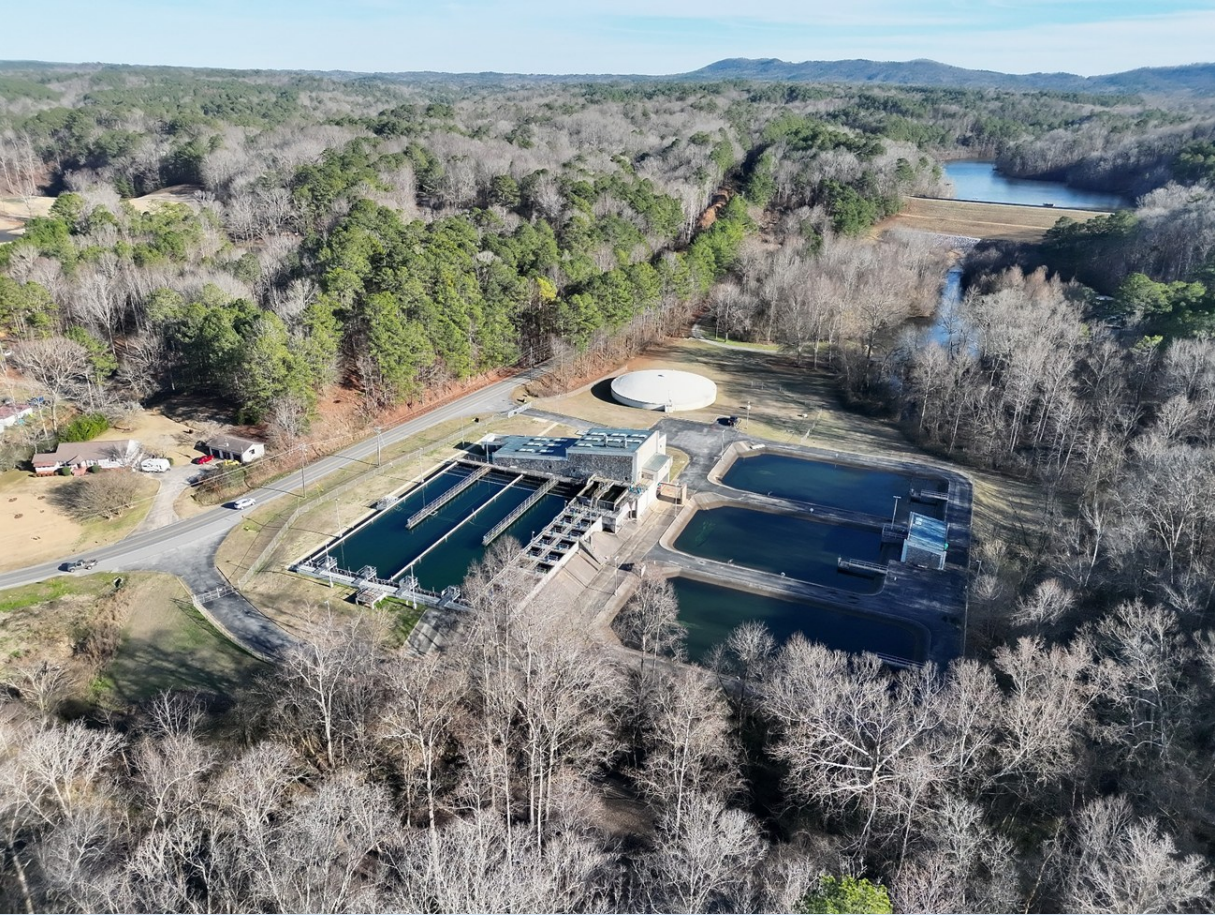
Knowlton Water Treatment Plant
